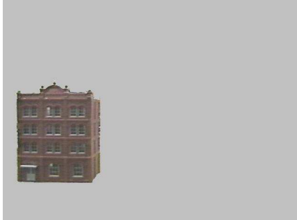
(b) The building
